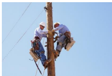
Figure 5.8: Dixie power employees and maintenance of area power lines.
