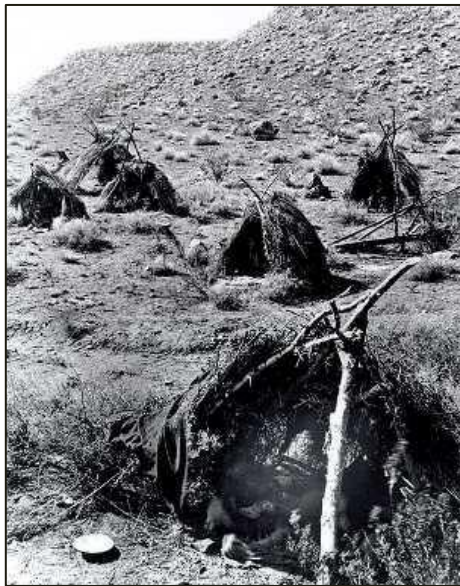
Figure 3.2: Ancestral Paiute wickiup dwelling in Iron County.
